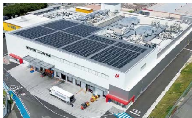
Exterior of new plant
