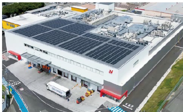
Exterior of new plant
